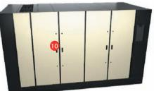
Hinged-door service access with integrated handles provides quick, easy access to all user-maintainable components—including the heat exchangers, which don't require removal during routine cleaning
